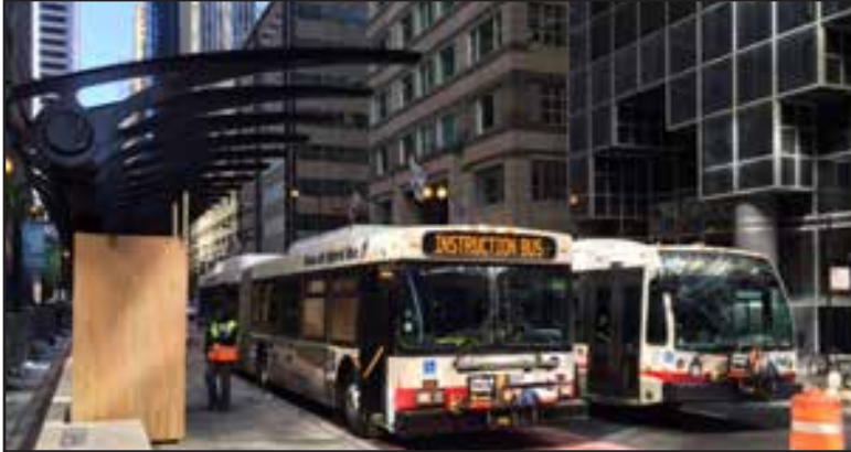
Construction to create distinct bus lanes, raised bus station platforms and more was ongoing in 2015 in downtown Chicago.
