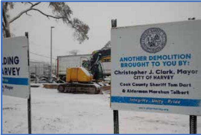
RENEW demolition site in Harvey
