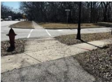
1st Avenue and Parkview Road. FPOC pathway in foreground transitioning to sidewalk opposite.
