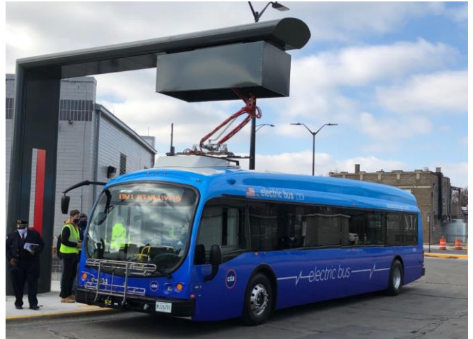
A new CTA electric bus uses the high-powered overhead charger at the Chicago Ave / Austin Blvd bus-turnaround
