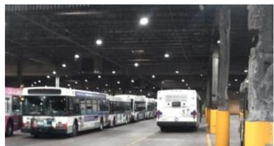
New LED lighting at CTA’s Chicago Bus Garage
