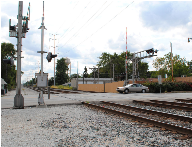
31 st Street west of Kenman Avenue
