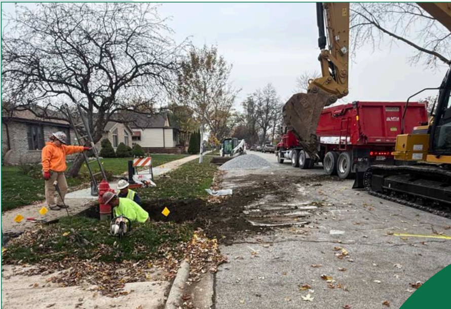
Priority community hydrant replacement during construction
