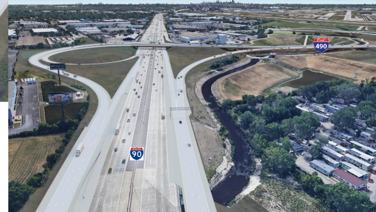
C) I-90 at I-490 – Looking East
