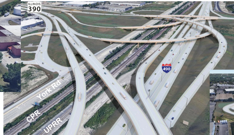
B) IL 390 at I-490 – Looking North
