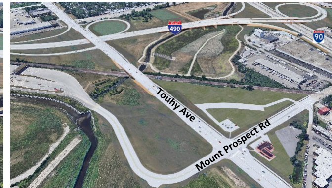
Realignment of Mt Prospect Rd - Looking West
