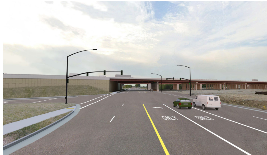
Franklin Avenue – Looking West
