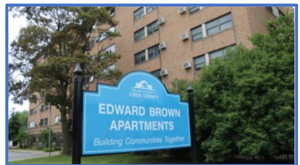
HACC Affordable Housing: South Suburban Senior Living, completed Nov 2019
