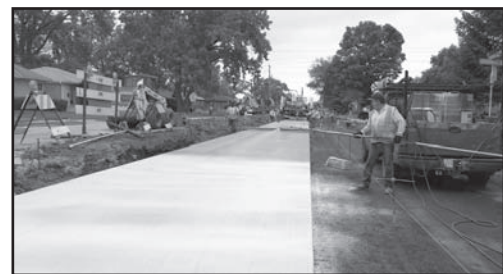
Concrete pavement construction on Crawford Ave.
