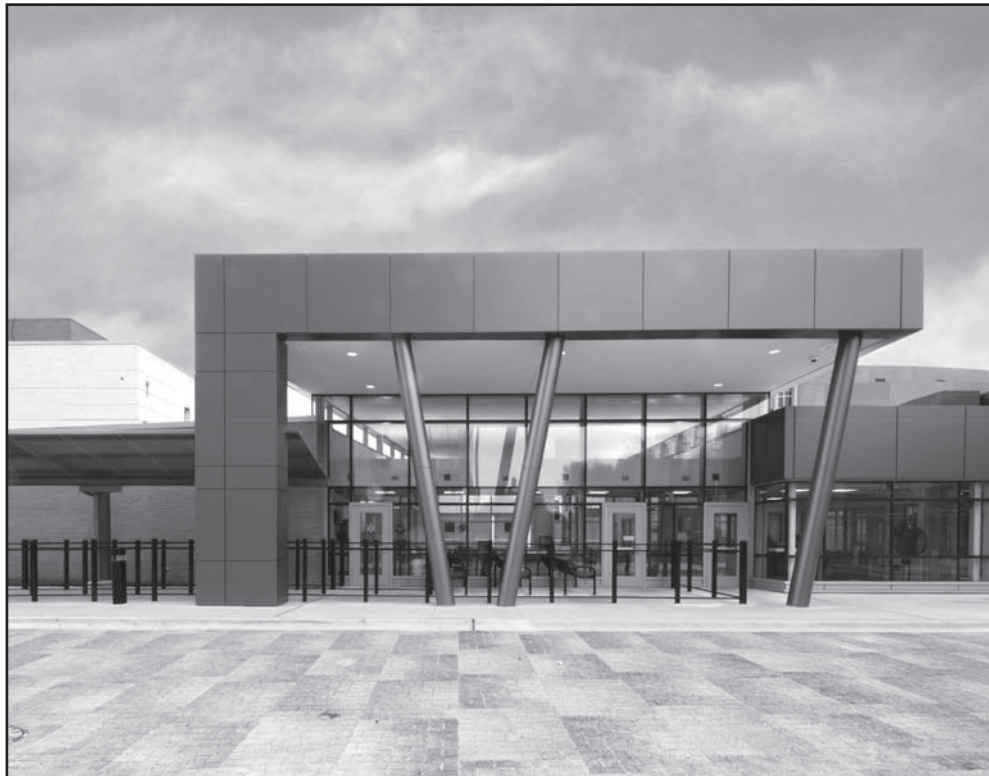
Department of Corrections – New Security Post
