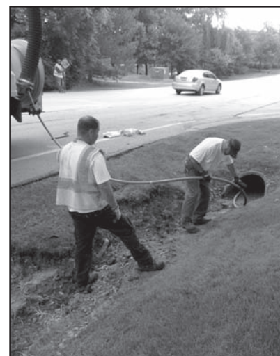
Culvert maintenance.
