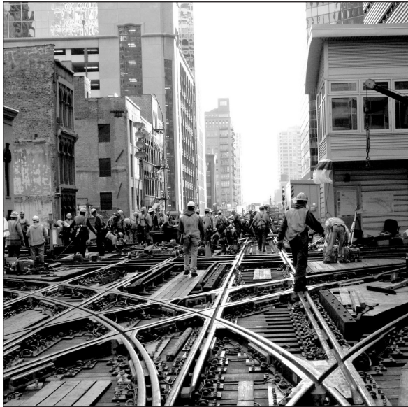
Crews worked around the clock over the course of four weekends to replace deteriorated rail ties and track components at one of the busiest rail junctions in the U.S. – CTA's Tower 18 –located at Lake/Wells. Five of CTA's eight rail lines travel through this junction each weekday.
