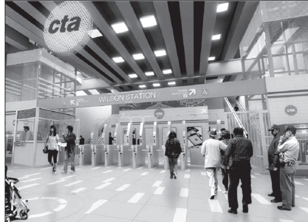
The completely rebuilt, modern and accessible Wilson station will provide new transit connections and serve as an anchor for revitalization and economic development in the Uptown neighborhood.
