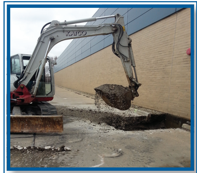
Pace is replacing the fire loop at its West Division garage.
