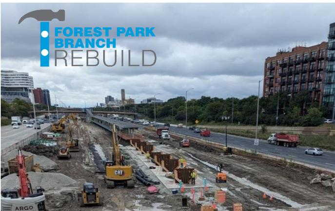
*Under Phase 1 of the Forest Park Branch Rebuild, crews completely removed and rebuilt nearly three miles of track bed along the Blue Line branch. Work also includes upgrading the power and signal systems and completely reconstructing the Racine station.*
