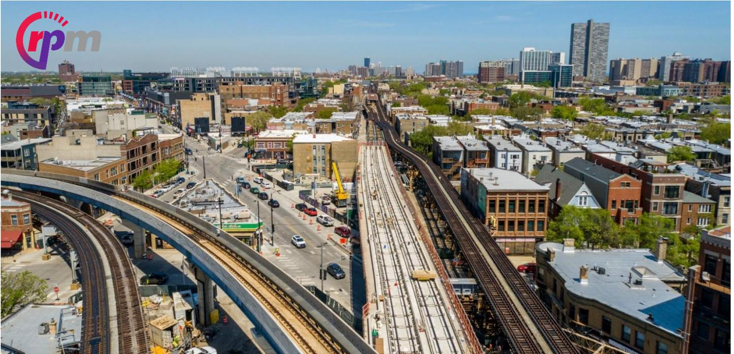
*Work associated with Red and Purple Modernization Phase One project continues. Aerial view of the final major stage of the Belmont Red-Purple Reconstruction project to straighten and remove a curve in the tracks to allow trains to move faster between Belmont and Addison.*
