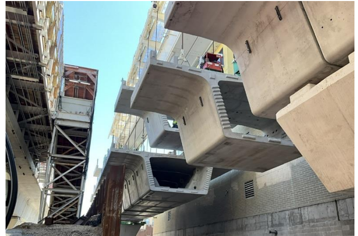
Pre-cast segments hang in place before being permanently sealed together to make a portion of the new elevated structure being constructed as part of RPM Phase One work.
